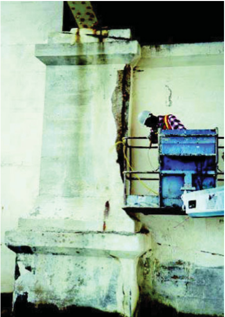
Figure 9: Typical condition of bascule piers.
