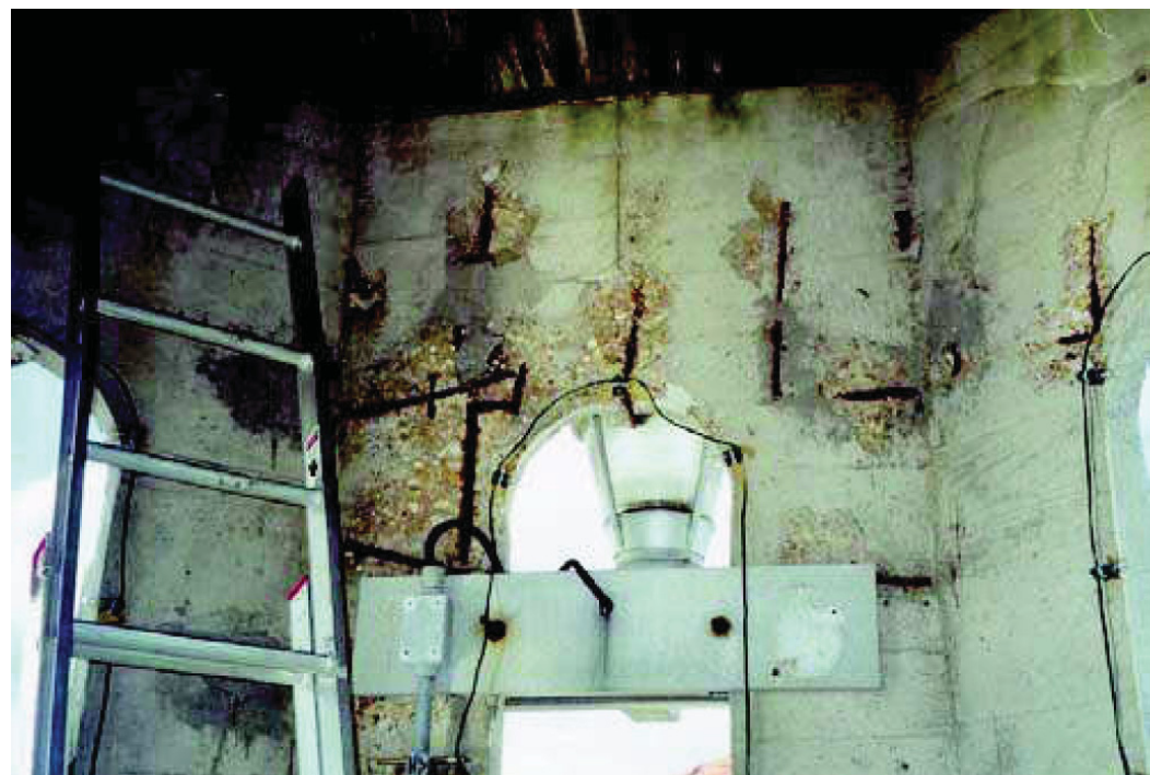
Figure 5: Typical condition of interior of towers where windows have been left uncovered.
