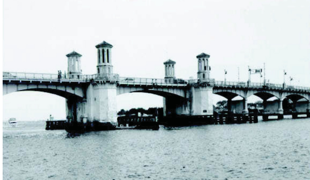
Figure 6: Elevation of existing bridge. Note arched girders and open approach pier configuration.
